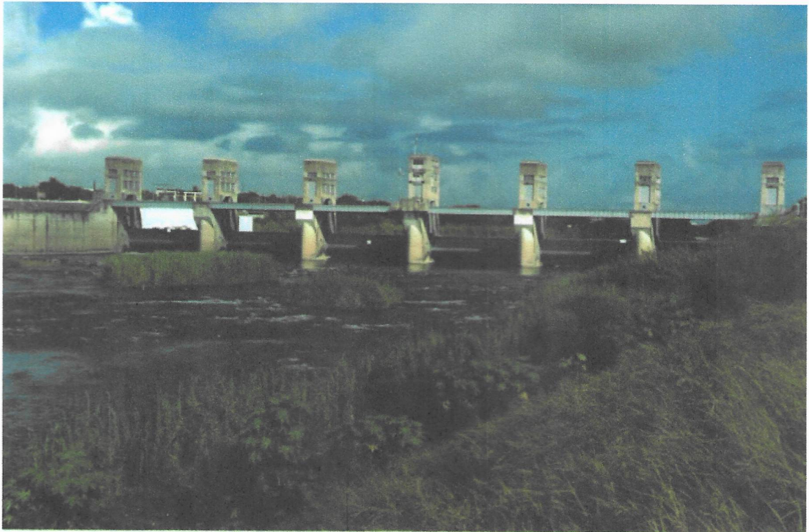
Figure 2. Anzalduas Dam, Mission, TX
