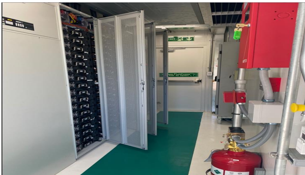
Figure 61. -An image of Novec fire suppression system as secondary fire control in energy storage system.
