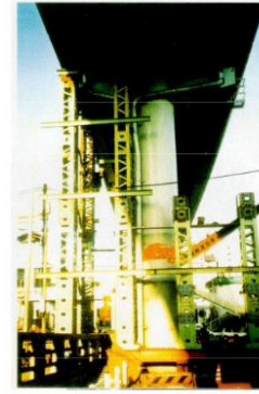
(b) Local buckling (circular section)
