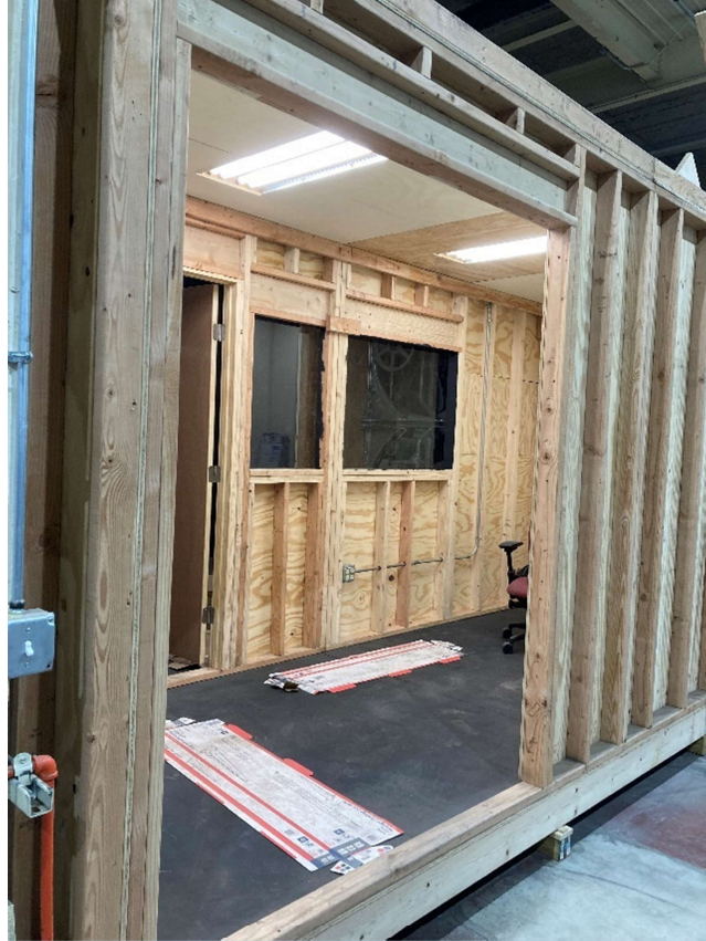
Figure 18. Test Section Control Room
