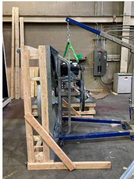
Figure 25. Fan and Cart Assembly with Mounted Motor and Flywheel
