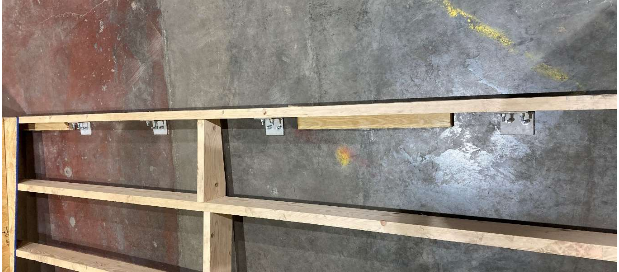
Figure 27. Mounted Brackets into Concrete
