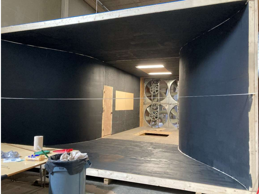
Figure 17. Constructed Inlet Contraction
