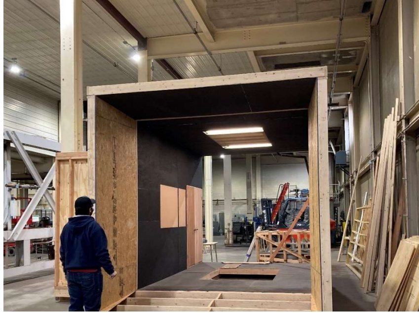
Figure 19. Constructed Test Section
