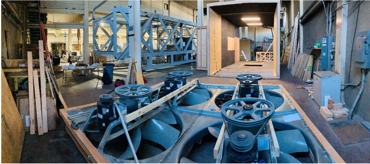
Figure 26. Constructed Fan Assembly prior to Lift
