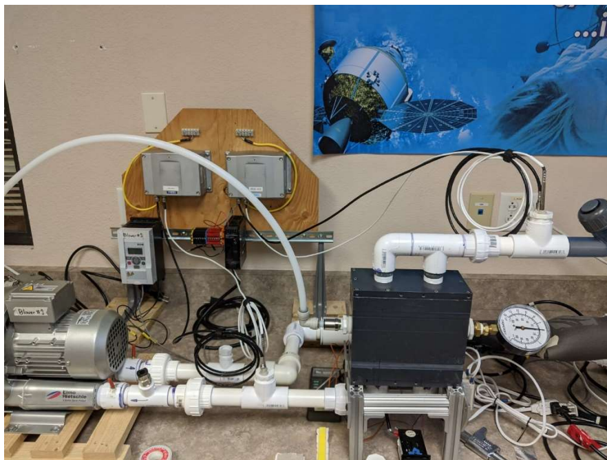
Figure 13. Added Relative Humidity and Temperature Sensors
