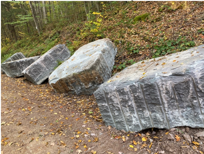
Image 2: Blocks utilized for base stone of rockery wall at Site 1 at Worlds End State Park
