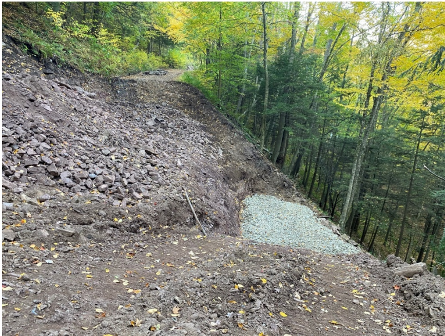
Image 1: Footprint of rockery wall with placed AASHTO No. 8 coarse aggregate at Site 1 at Worlds End State Park
