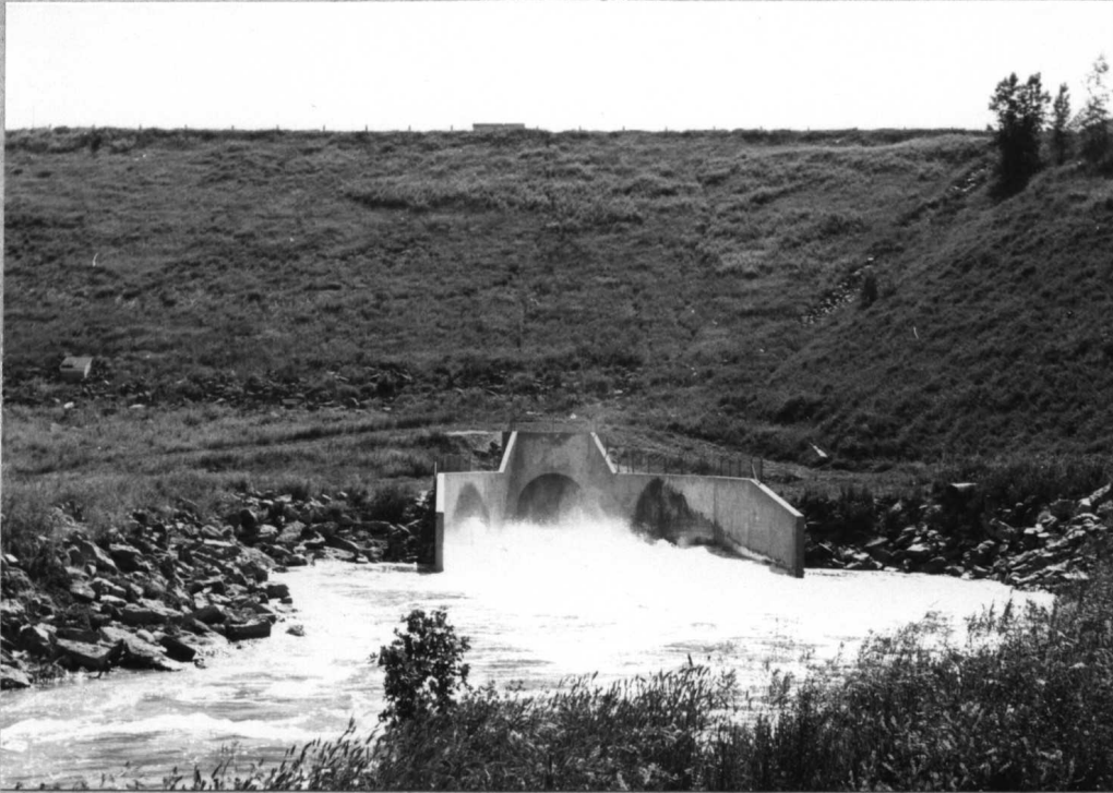
Fig. 18.--Heart Butte Dam and tail race outlet area.
