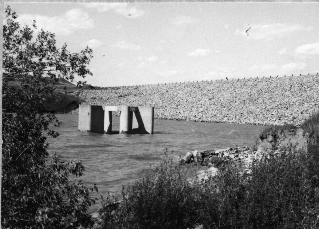
Fig. 17.--Heart Butte Dam and intake structure.
