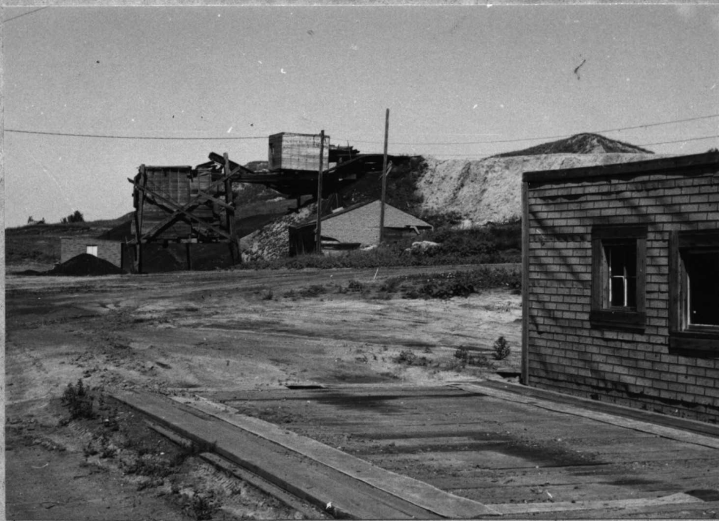
Fig. 29.--Loading and weighing facilities at Davenport Mine.
