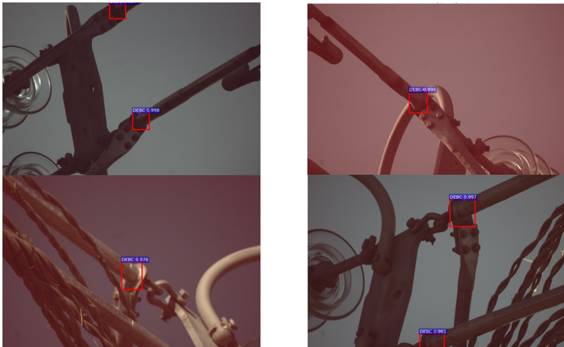
Figure 20: Example results of successful DEBC detections.
