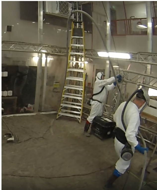
Figure 57. Air umbilical being suspended from pulley system and tied off.
