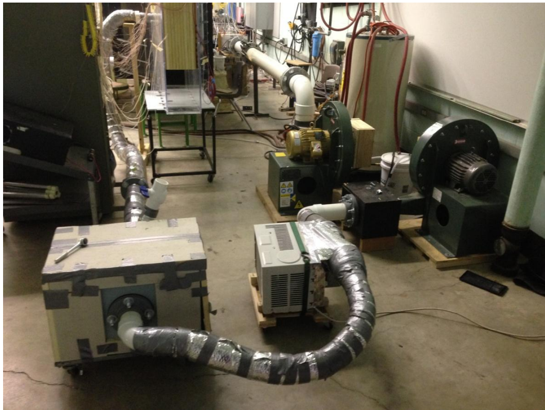
Figure 25. Entire coolant supply system.
