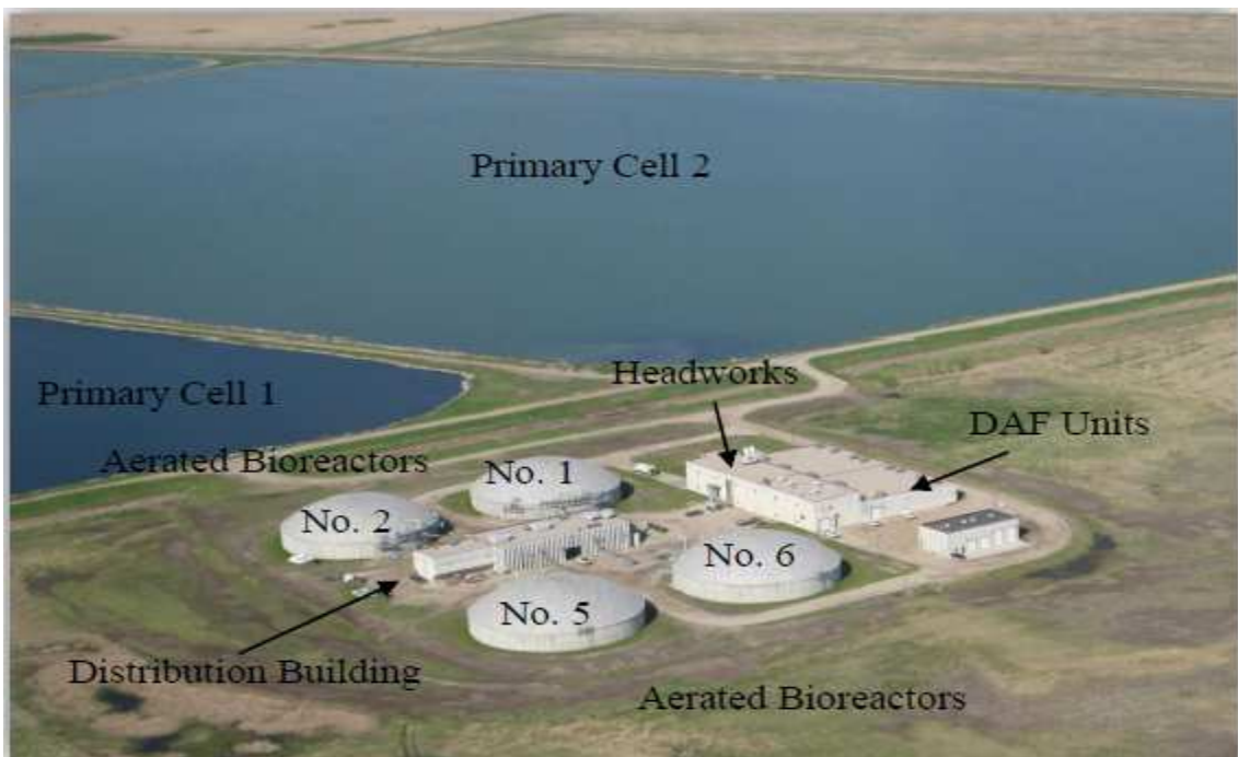
Figure 2-1: Aerial Photo of GFWWTP
