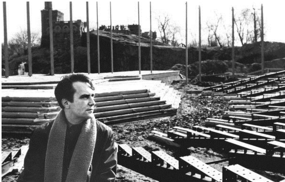
Picture of Joseph Papp during construction of the Delacorte Theatre (Grove)
