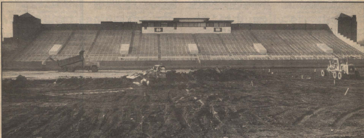
Preparing Memorial Stadium for artificial turf.
