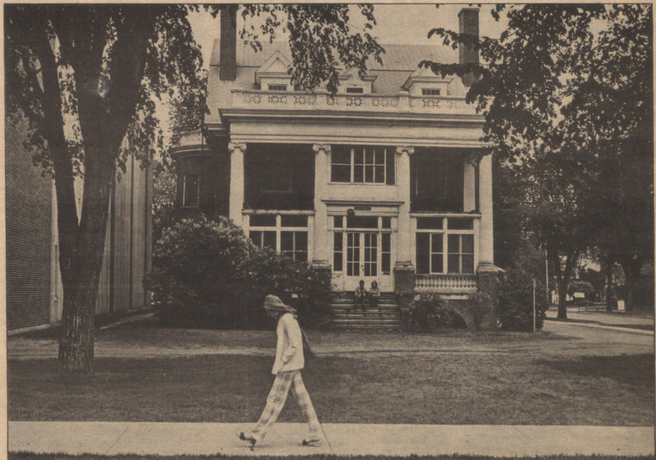
Oxford House, located just 18 feet north of Gamble Hall, once was destined for the wrecking ball. Now the 77-year-old former president's residence is scheduled for renovation and continued use as the University's visitor's center and as home of the UND Alumni Association and Foundation.
