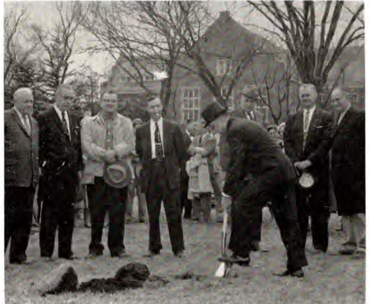
This was the historic moment when ground was first broken for the campus' new $1,000,000 Chester Fritz Library. President Starcher is shown turning the first sod. Looking on, are Architect Theodore Wells, State Board Member Fred Orth, Contractor Walter Johnson, Librarian Donald J. Pearce, Business Manager, E. W. Olson, Alumni Director J. Lloyd Stone and Alumni President Loyde Thompson. In the background is the present library.
