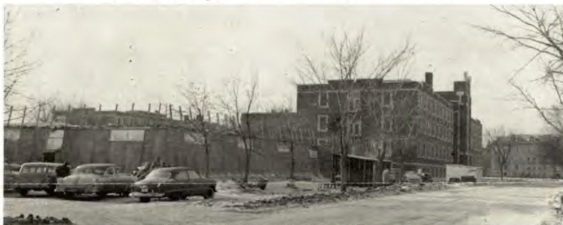
This view, looking west along Second Avenue North, shows the location of the new Rehabilitation Center in relation to the Medical Science Building, at the right of the picture. Brickwork now is in progress on the Rehab building, under the canvas shroud installed to keep out wintry blasts. When completed, the $300,000 facility will be of Gothic design to match other campus buildings.
