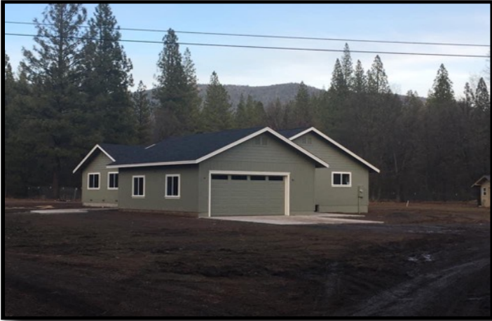
Brad and Alicia's house days after my father completed it. Photo credit: Alicia Dalton.
