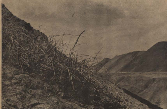
Sod on a spoil pile—evidence, say miners, that NACCO isn't obeying the state's strip mine reclamation law which requires segregation of topsoil.
