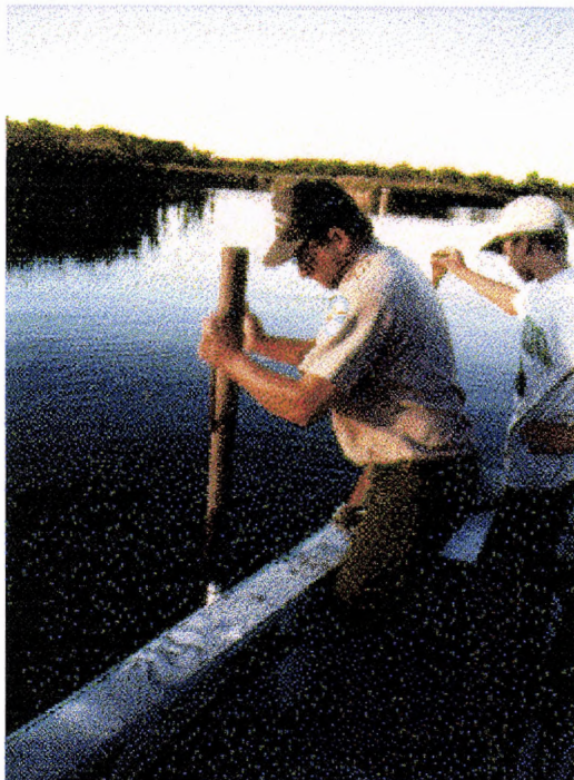
Figure 11. Henry Duray (Icelandic State Park Manager) and Andrew Duray helping to install piezometers.
