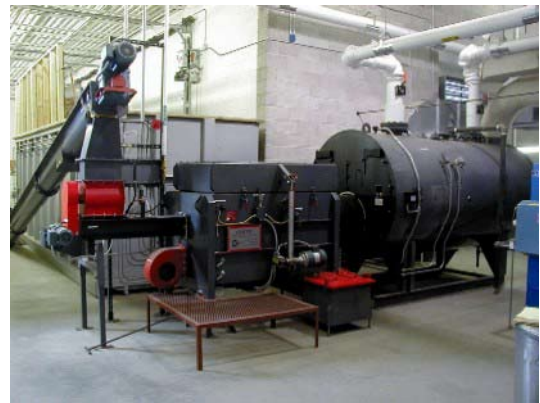
Figure 2. Example of a wood heating system ( www.chiptec.com ).
