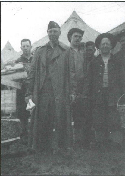
Lt. Geston and members of C Company building a board walk in company area, Camp Claiborne, LA - 1941.
