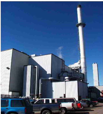
University of North Dakota steam facility.
